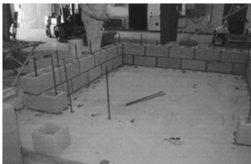
Fig. 6. Shelter walls dowels
