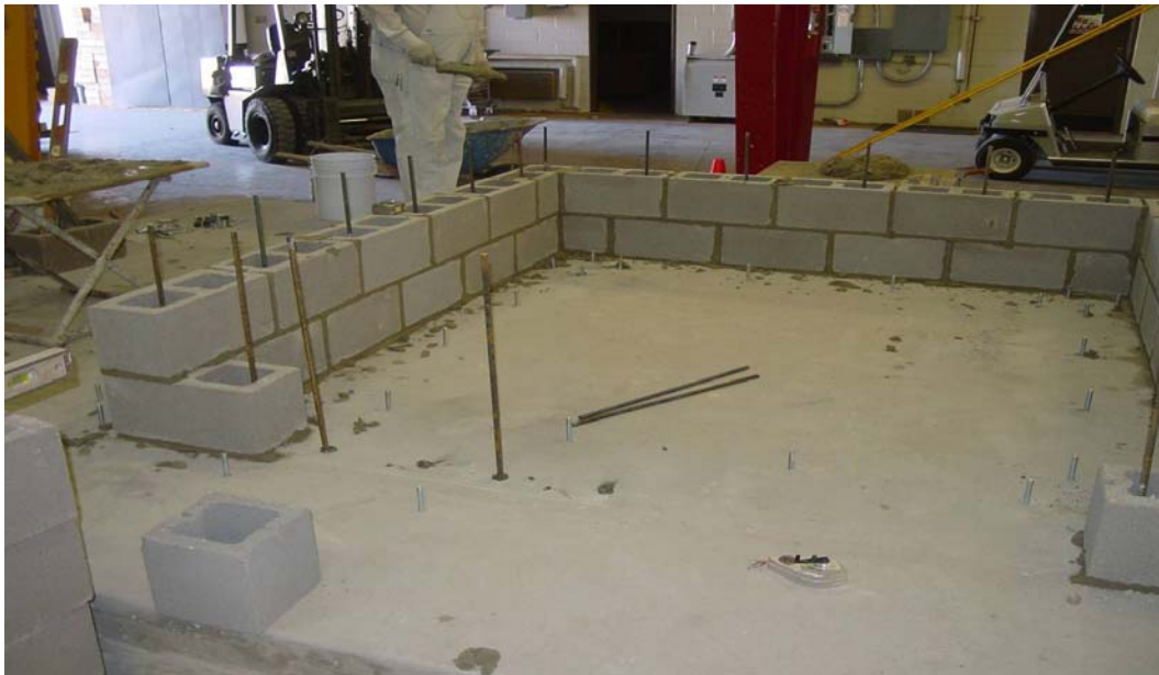
Fig. 7 - Reinforcement within shelter walls
