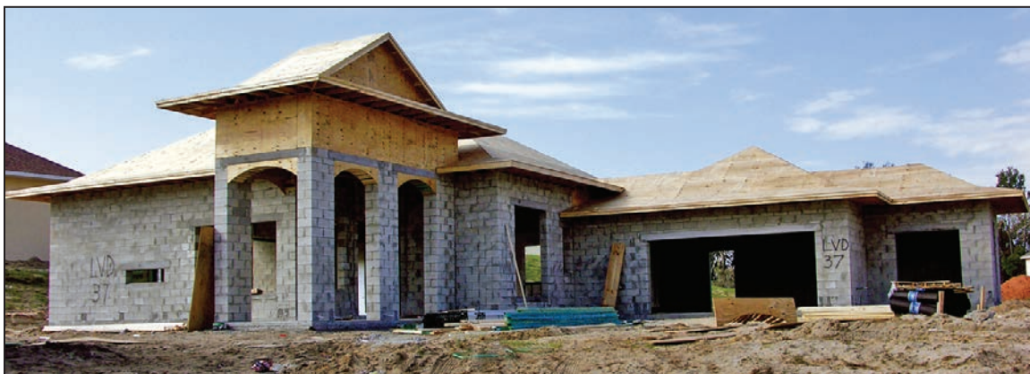
Figure 3-3: Exterior walls constructed of CMU (New Smyrna Beach, FL, 2007)
